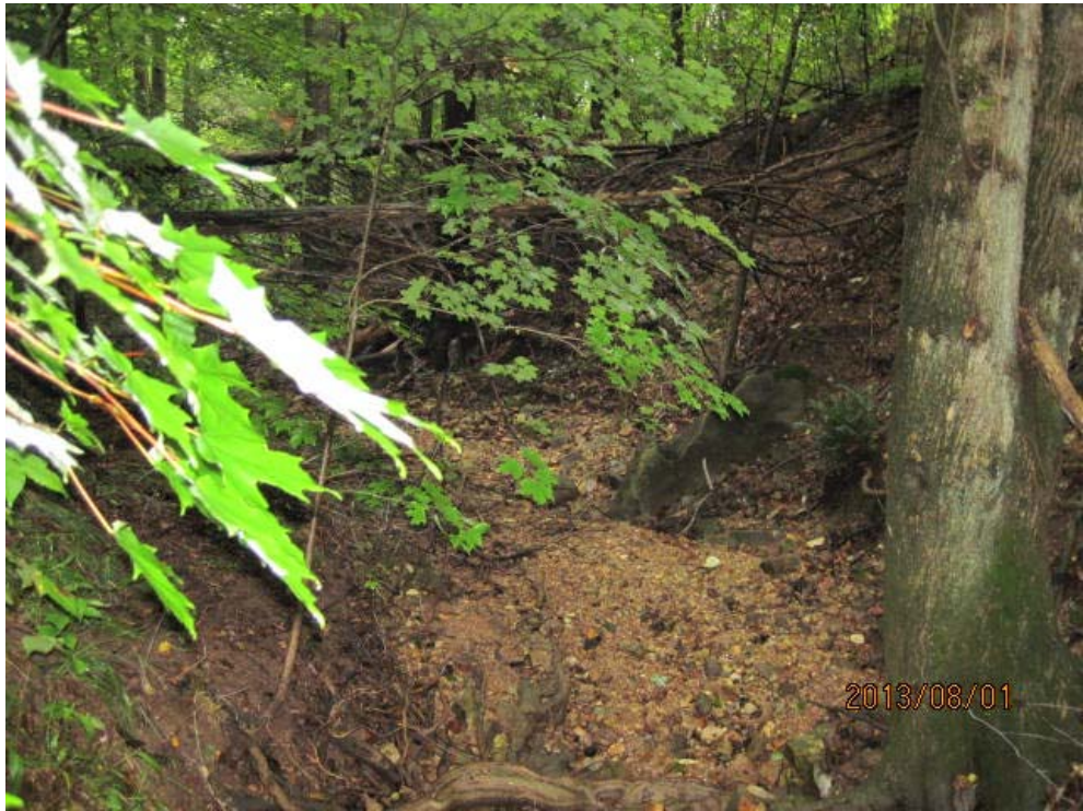
Photo 5. Downstream view of STR-1 at Sta. 733+40L.
