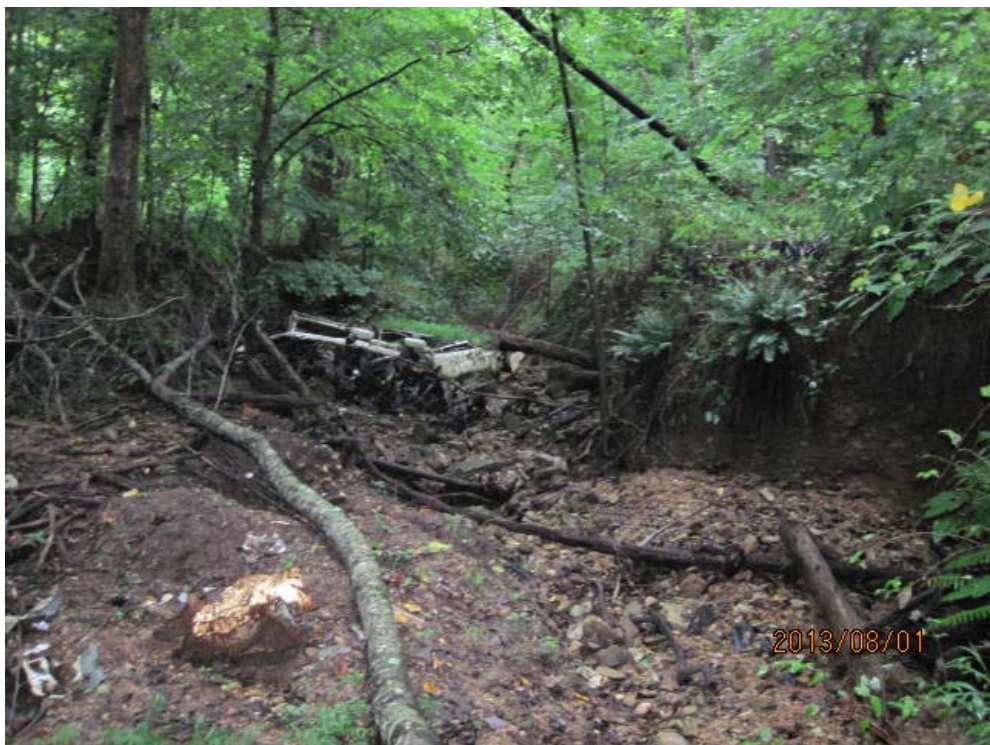
Photo 6. Upstream view of STR-1 at Sta. 733+40L.
