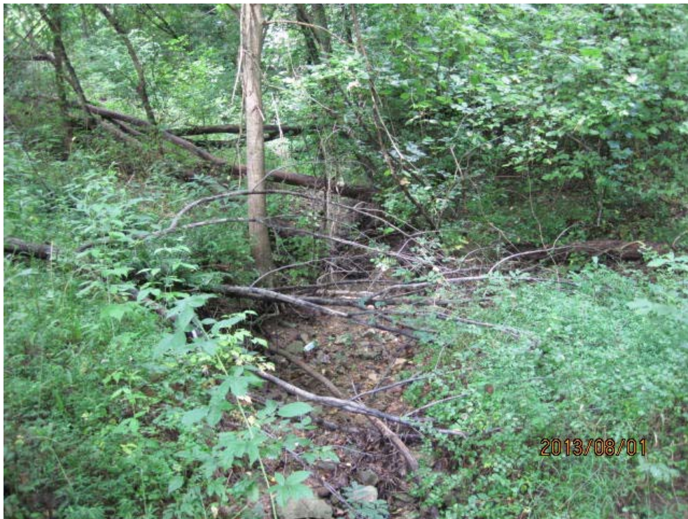
Photo 4. Upstream view of STR-1 at Sta. 725+00L.
