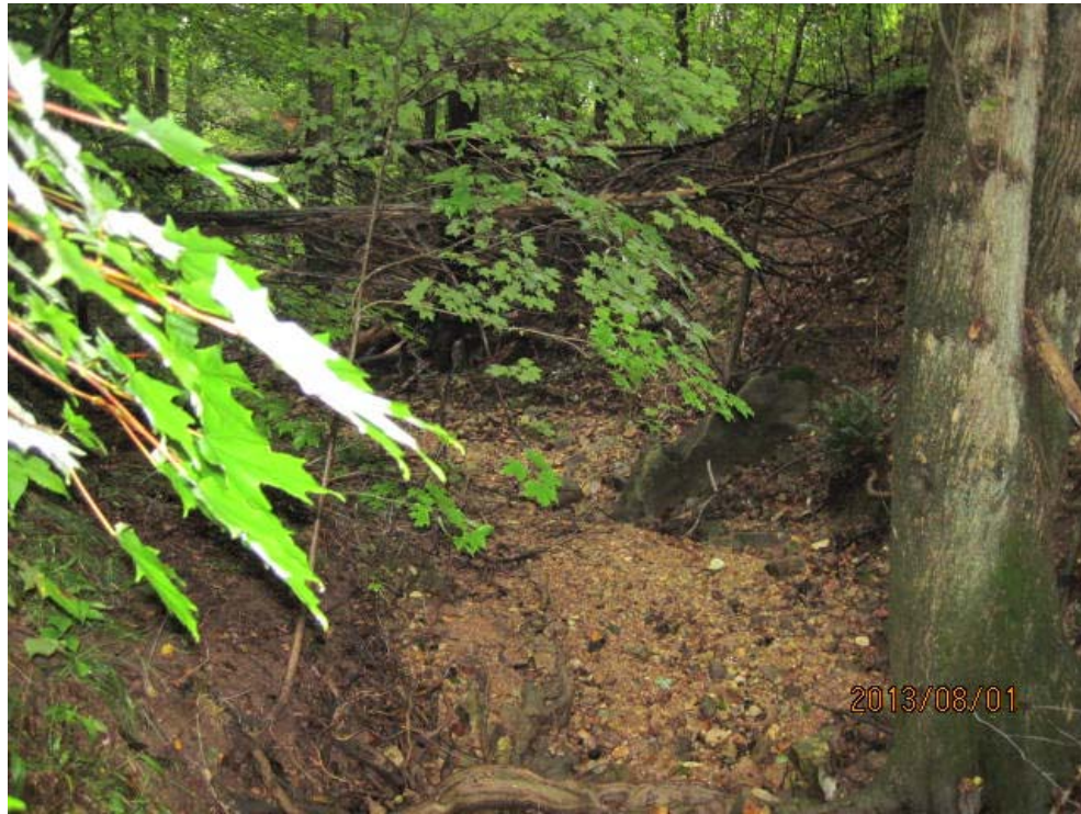
Photo 5. Down-gradient view of WWC-2/EPH STR-2 at Sta. 733+40L.
