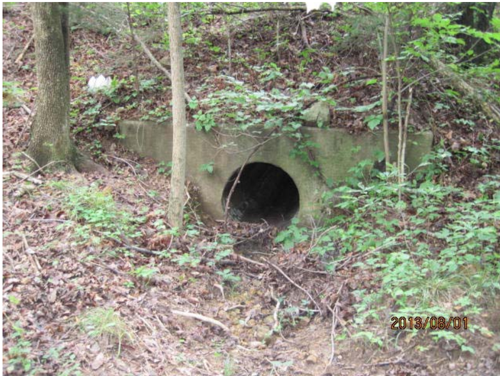
Photo 2. Down gradient view of WWC-1 toward culvert inlet.
