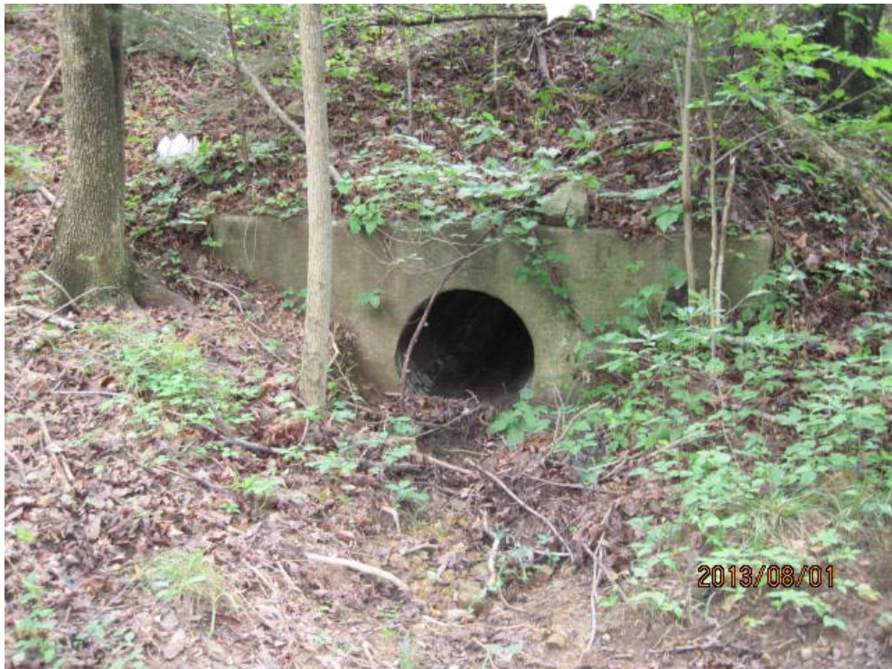
Photo 2. Down gradient view of WWC-1/EPH STR- 1 towards culvert inlet. 1
